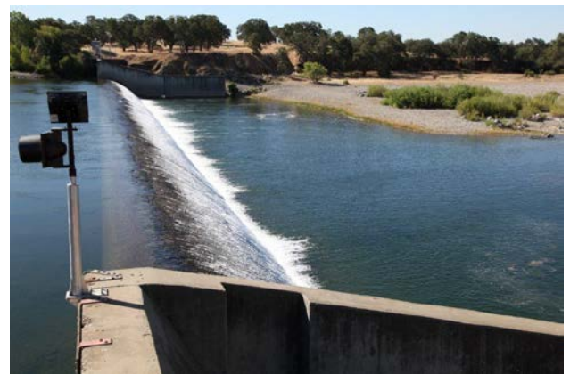
Figure 1-6. Daguerre Point Dam.
