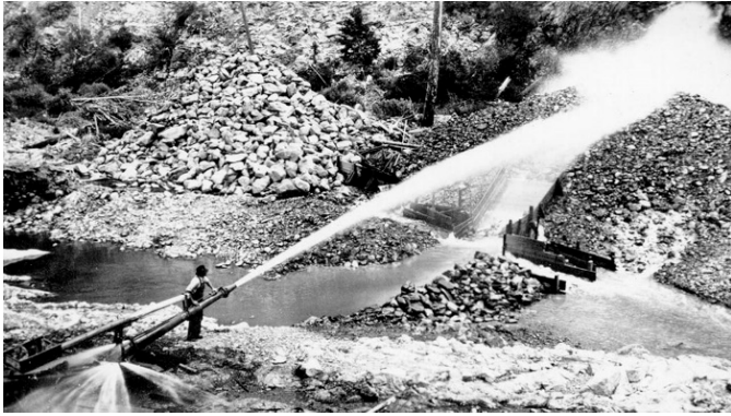
Figure 1-1. Hydraulic miner operates a water cannon.
