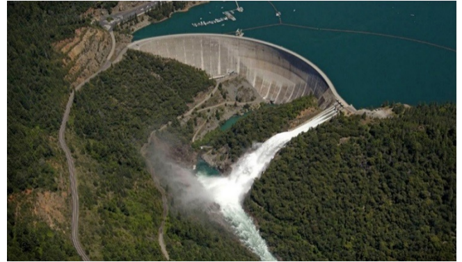
Figure 1-8. New Bullards Bar Dam.
